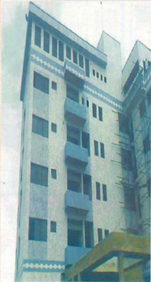
8 STOREY HOTEL BUILDING FOR AKFAT HOTELS AND TOWER IWO ROAD, MONATAN, IBADAN, OYO STATE
