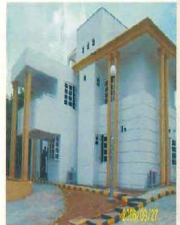
OSUN STATE GOVERNOR'S HOUSE AT ASOKORO, ABUJA, FCT.
