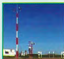
Automatic Weather Observation Systems
